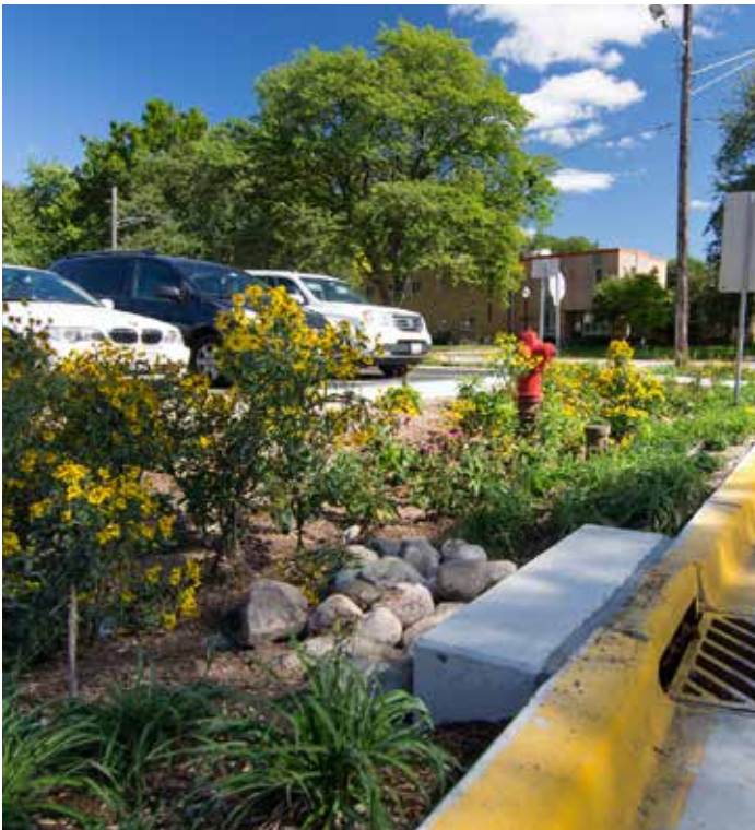
Stormwater runoff from a parking lot is delivered to a series of rain gardens to reduce runoff (CNT)
