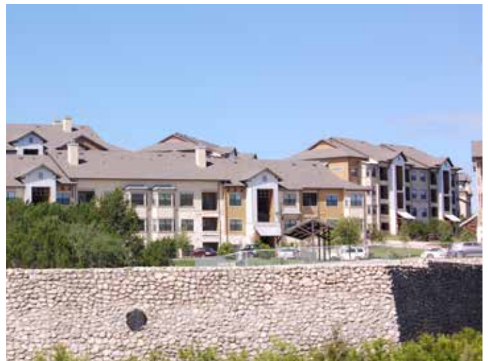
Multi-family housing under construction
