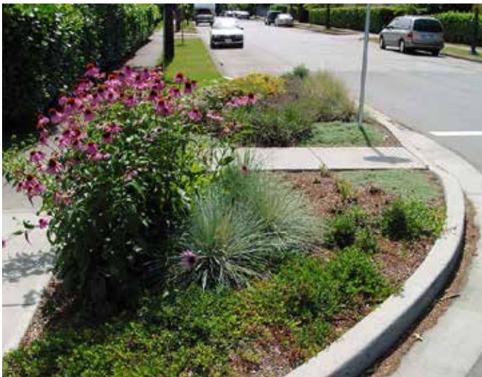
Landscaped curb extension in a residential neighborhood helps to slow traffic and improve neighborhood aesthetics (Richard Drdul, Flickr Creative Commons)
