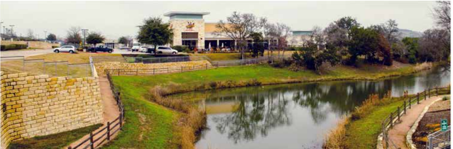
Water feature provides a dual purpose: stormwater management and a natural amenity along the Hill Country Galleria Trail
